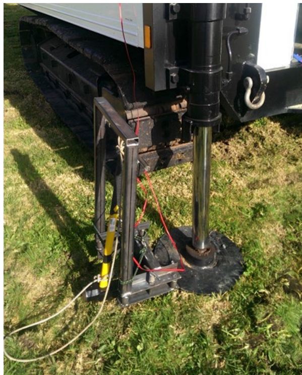
Figure 1: Seismic CPT in action
